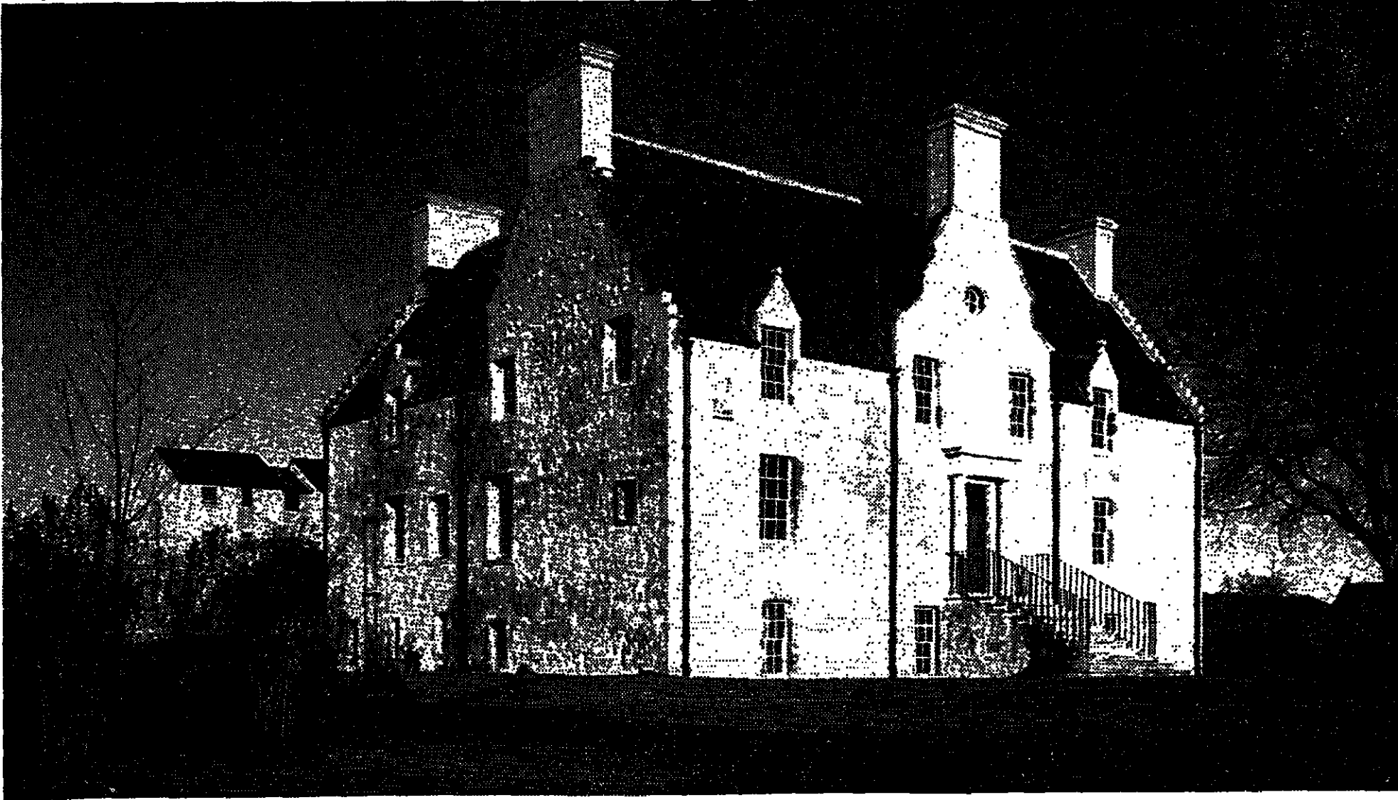
Pirlig House, built 1638. Burnt down, 1971. Restored by Wimpey Homes and Michael Laird & Partners, architects, 1986.
